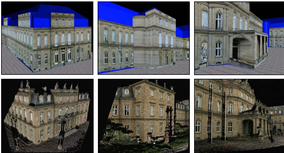
Fig. 6: Available architecture model of the Stuttgart palace from aerial images improved by manual texture mapping (top) and 3D point clouds acquired automatically with the proposed trifocal sensor system using one image triplet (bottom).
